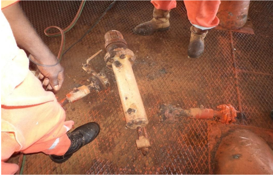
A BAD CORRODED LEVEL SWITCH DISMANTLED FOR REPLACEMENT OF A NEW ONE
