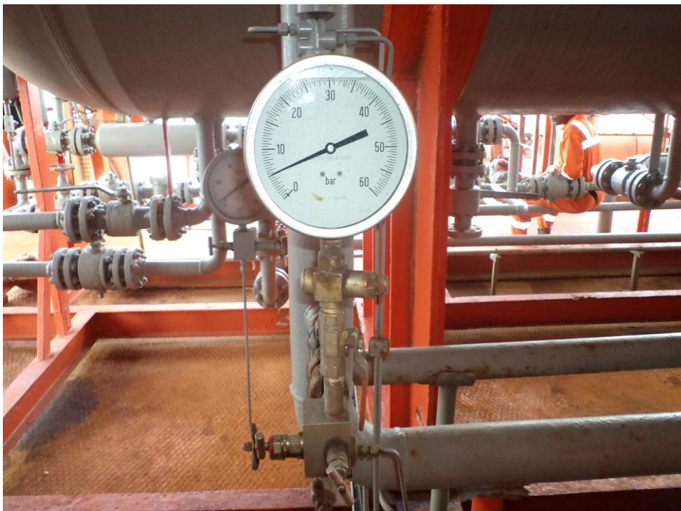
COMMISSIONING OF A PRESSURE GAUGE AFTER INSTALLATION
