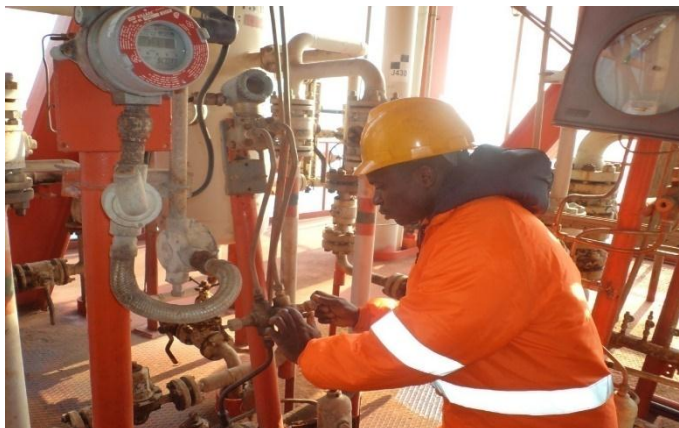
PURGING OF A DIFFERENTIAL PRESSURE TRANSMITTER AFTER AN ON-LINE CALIBRATION
