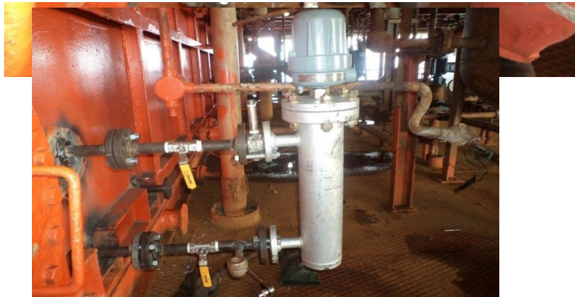
COMMISSIONING AFTER FABRICATION AND PRESSURE TESTING THE JOINTS.
