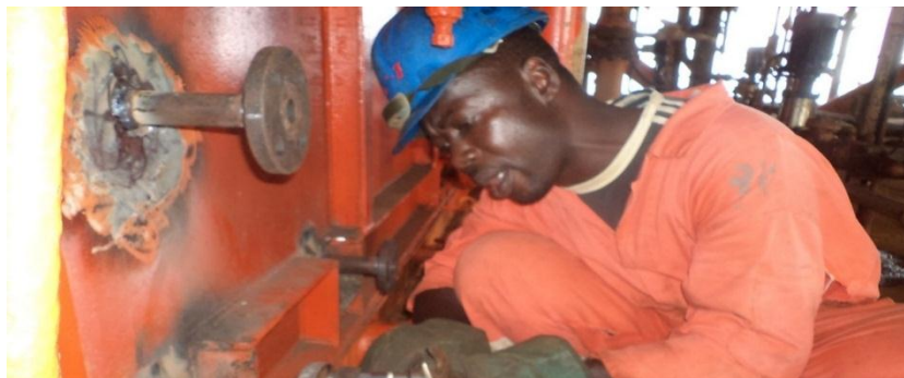
COUPLING OF FABRICATED SPOONS AND MANUAL VALVES FOR THE INSTALLATION OF A NEW LEVEL SWITCH
