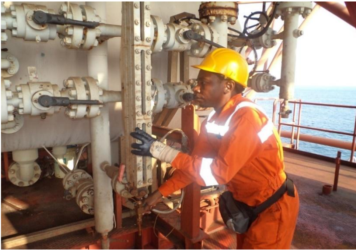
TAKING THE LIQUID LEVEL OF A LOW PRESSURE SEPARATOR AFTER THE CALIBRATION OF IT'S LEVEL SWITCH
