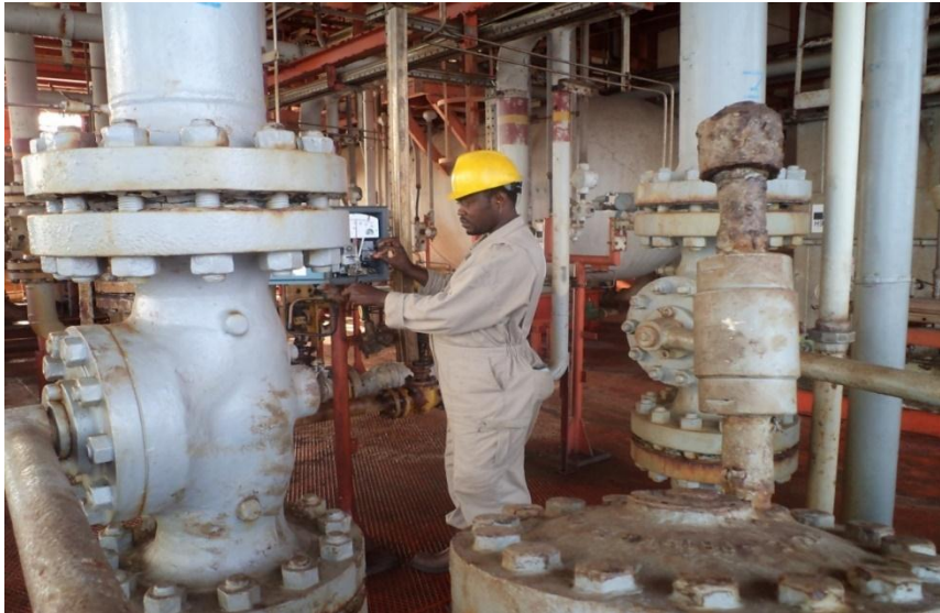
ADJUSTING THE SET POINT OF A PIC (PRESSURE INDICATING CONTROLLER) BENCH CALIBRATION AND INSTALLATION
