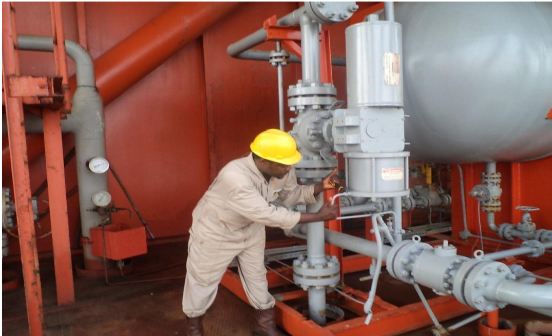
CONNECTING AN INSTRUMENT AIR SUPPLY LINE TO A SHORT DOWN VALVE READY FOR COMMISSIONING
